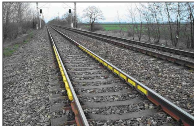
Fig.2. Dynamic scale and flat spot detection of Austrian Federal Railways (Infrastruktur Betrieb AG)
